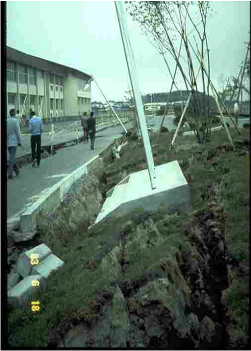
Figure 1.2 1983 Nihonkai-Chubu: Liquefaction caused unstable soils to fail. Flagpole foundation foreground was placed shallowly. School building to the left was founded on a pile foundation and suffered no damage.
