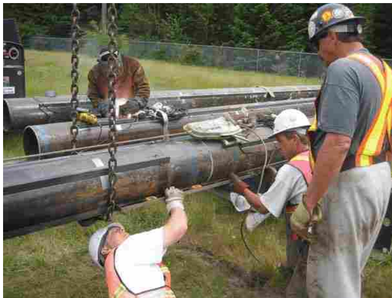
Figure 5.8 Welding the instrumented segments of the test piles before driving.
