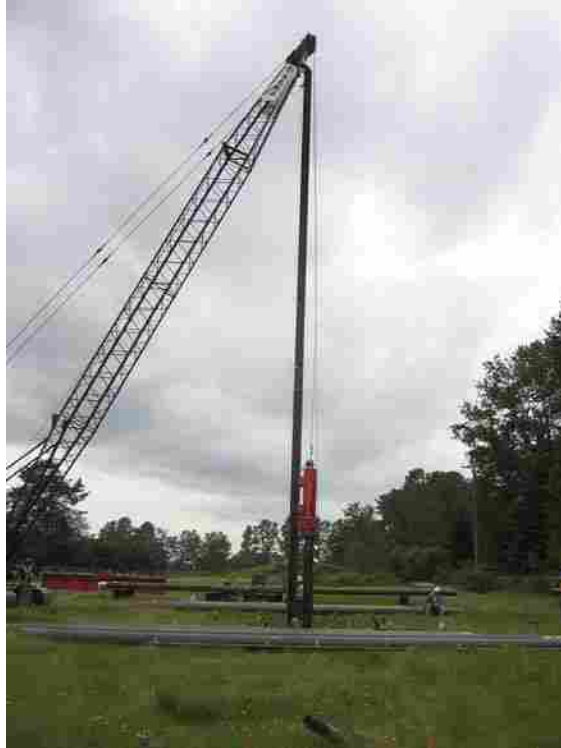
Figure 5.9 Photograph of test pile being driven with 2500 kg drop hammer.
