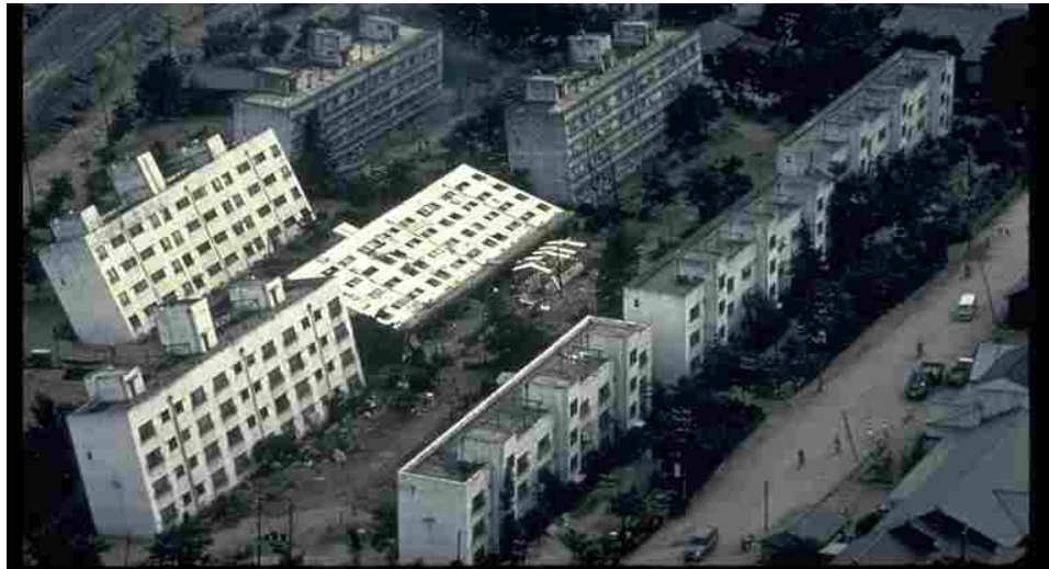
Figure 1.3 1964 Niigata Japan: Liquefaction caused major settlement. The building at center rotated 70 degrees from vertical. Surprisingly, little structural damage occurred to the apartment buildings. Some buildings were later righted and re-inhabited.
