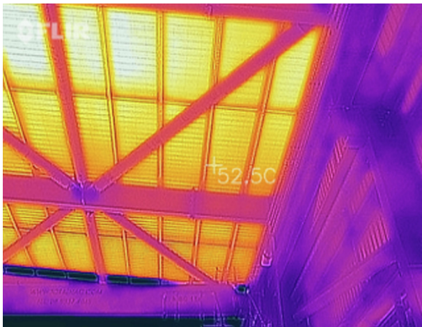
Fig. 9. Roof of one of the mill sheds, at 52.5 °C.
