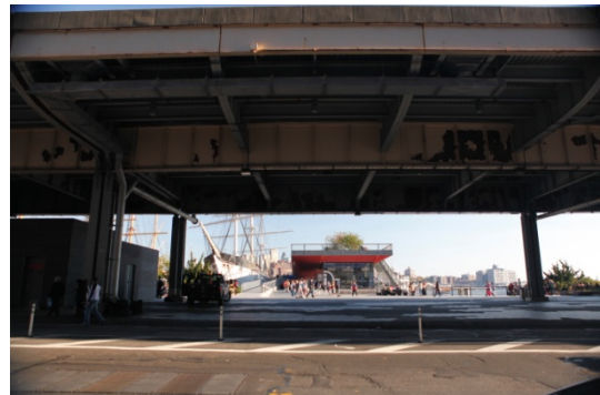
Figure 31 Under FDR Road in front of the Site
