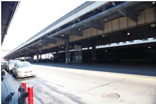
Figure 32 Existing Condition Under FDR Road
