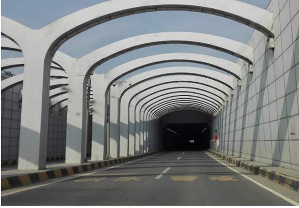
Fig. 1. Pergola at the portal of a tunnel.
